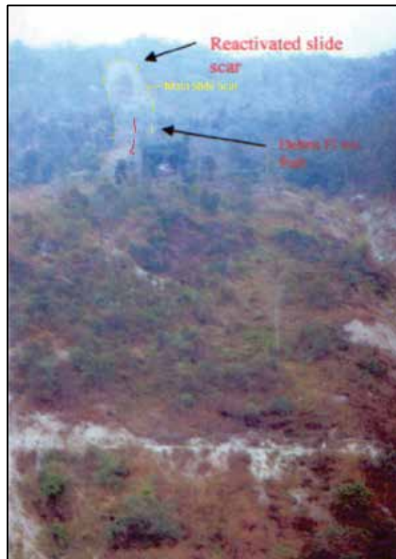
Photograph 2 Reactivation of slide with debris flow path from the main old slide scar above "Zone-C"
